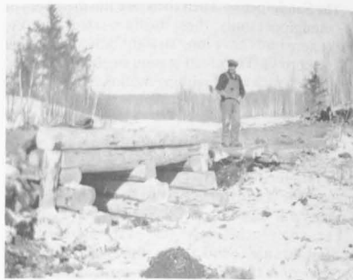
Construction of wooden culvert near Junction of Toniata Road and PR 301.
