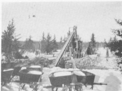
Wheelbarrows were used to take gravel to crusher, these were all hand loaded and moved to crusher by men.
