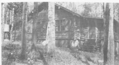
Bennett cottage with water barrel for gravity flows water to the tap in the kitchen.
