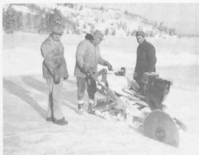
The biggest ice cutting operation in the area. Here Mr. Blackwell is marking off the ice in large squares with a circular ice-saw.
