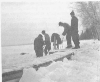
Adolph Zimmerman and helpers lifting blocks of ice from the water at Lakeside Cabins. From here they were taken by truck to the ice-house, stacked tightly together, then covered with many loads of sawdust, where it would last all summer.
