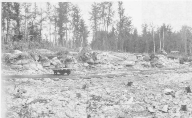
The crude tracks laid to move rock and gravel for road base.
