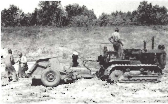
Photo 19. Mining a Bentonite Seam, Pembina Mountain Clays Limited, Morden Area. Today, the workmen would be wearing hard hats and the tractor would be equipped with a roll-over protective structure (MRD).
