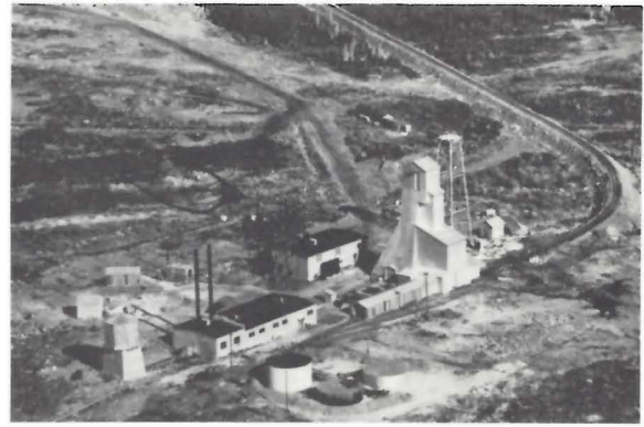
Photo 62. Surface Plant, EL Mine, Sherritt Gordon Mines Limited, Lynn Lake Area. The circle to the left of the headframe marks the stope break-through to surface (MED).
