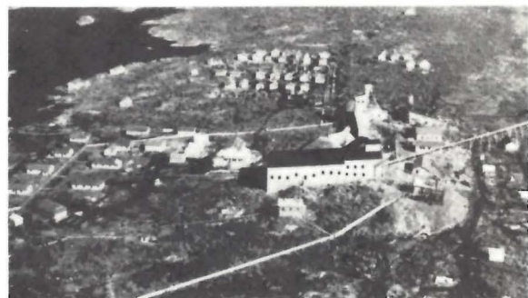
Photo 38. Surface Plant, God's Lake Mine and Townsite, God's Lake Mines Limited, Gods Lake, 1935 (RCAF).
