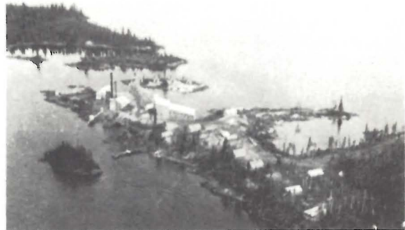
Photo 37. Surface Plant and Camp, Island Lake Mine, Island Lake Mines Limited, Island Lake (ca. 1934) (MRD).
