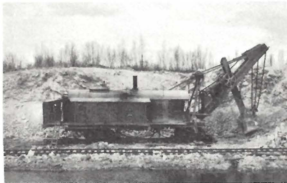
Photo 20. Quarrying Gypsum at Gypsumville, Manitoba Gypsum Company (ca. 1927) (MRD).
