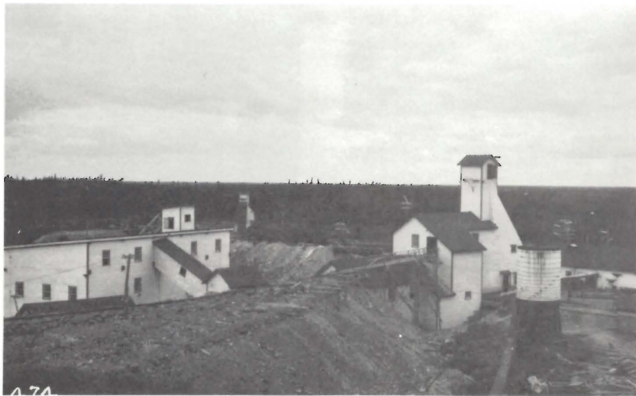
Photo 33. Surface Plant, Gunnar Mine, Gunnar Gold Mines Limited, Beresford Lake, 1935 (MRD).
