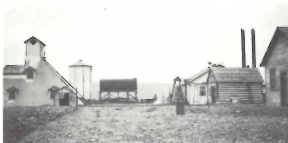
Photo 39. Surface Plant, Mandy Mine, Mandy Mining Company, Flin Flon Area, 1929. Manitoba's first base metal producer (MRD).
