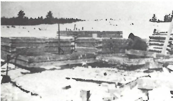
Photo 79. Framing Jack Nutt Shaft Timber by Hand, Bernic Lake, 1928 (TANCO).
