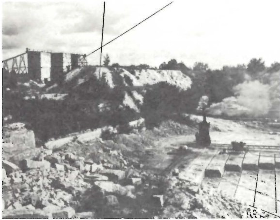
Photo 10. A study in the evolution of limestone quarrying: The Old — cutting channels by steam operated chisel-tipped hammer (MED).
