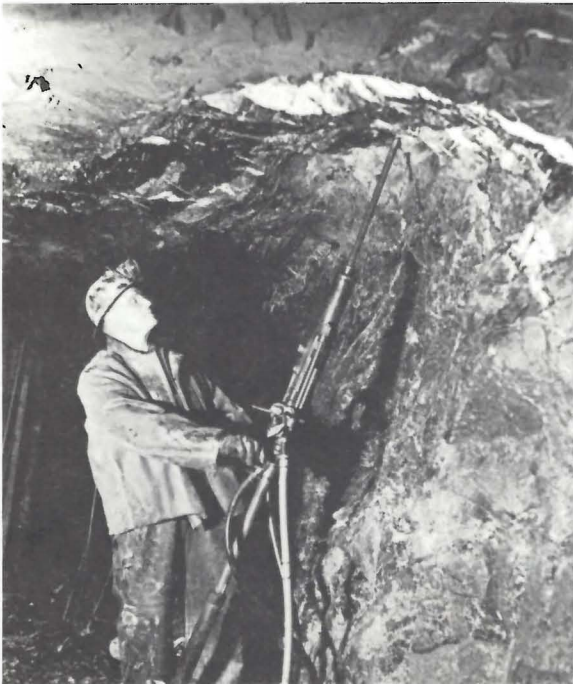
Photo 61. Drilling "Uppers" at a Lynn Lake Mine, Sherritt Gordon Mines Limited (SGM).
